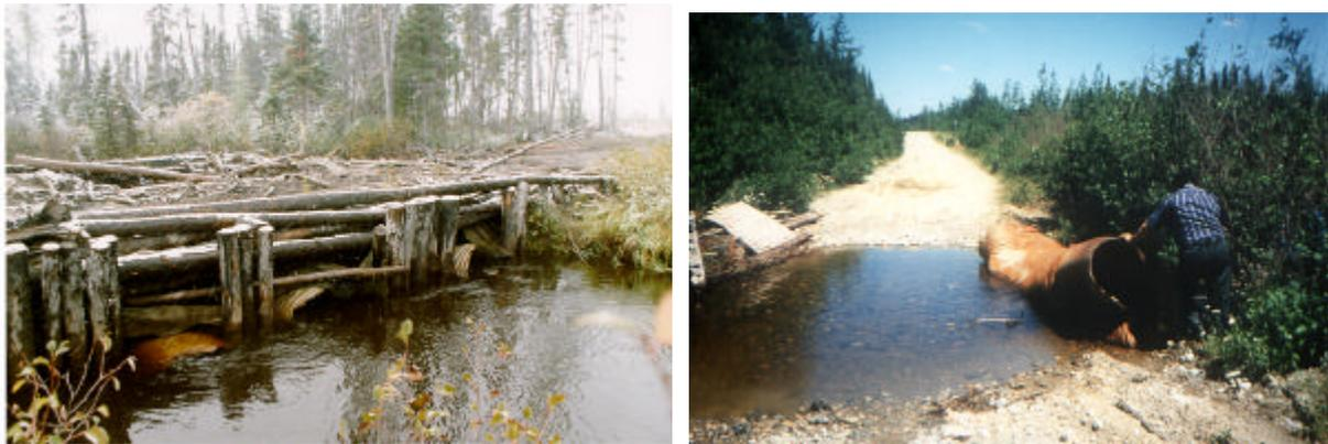
*Using metal drainage culverts instead of proper bridging material leads to flooding, soil erosion and washouts.*
